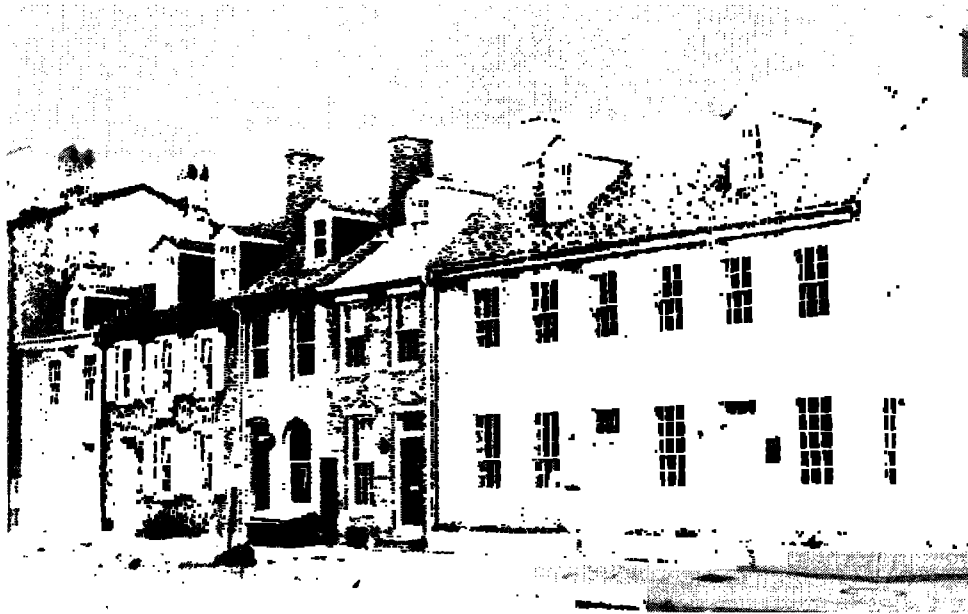
(a) 1-11 East Montgomery Street (1 is on the right)
